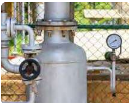
New flash vessel installation and condensate line resizing
