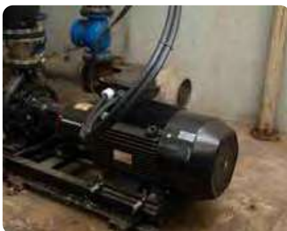
Energy efficient pump replacement at the wastewater treatment plant and effluent treatment plant
