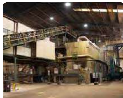
Smart Energy saving system for Stenter machines
