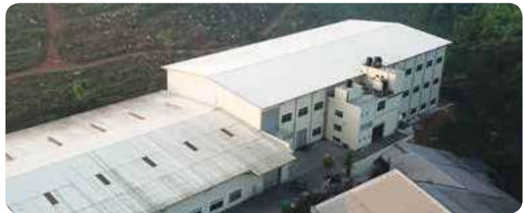
Establishment of the new knitting building
