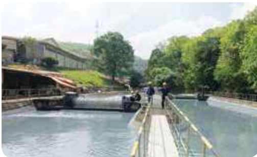
Effluent treatment plant
